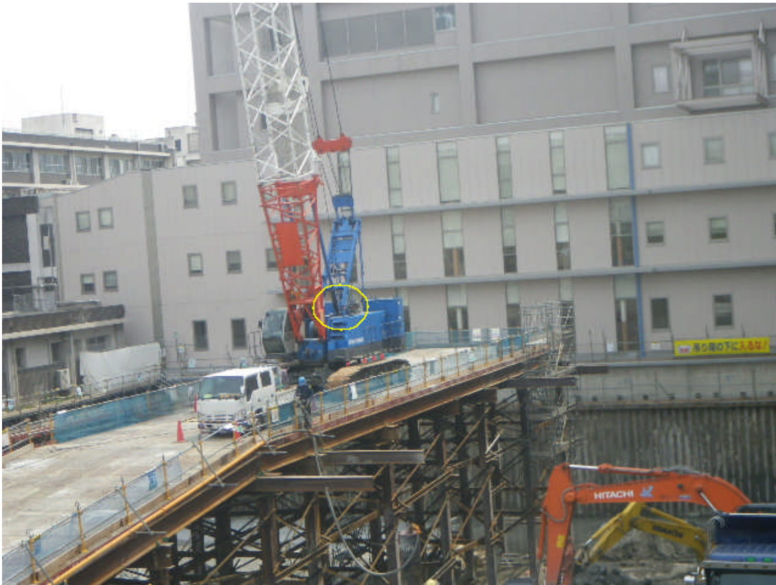
At a hospital construction site.
